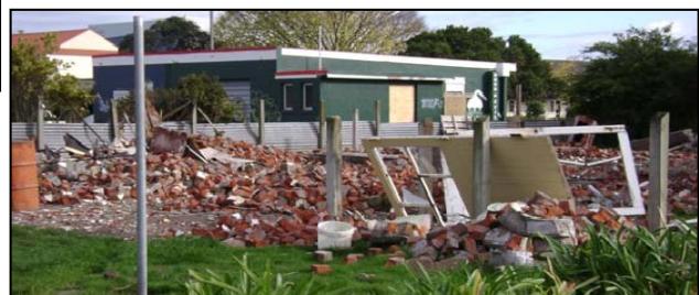
Corner Featherston & Ngata Streets, house removed and clean-up to be completed
